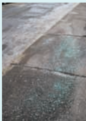
Figure 6.16 Some road salts contain colour to make it easier to see where they have been spread.
