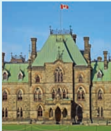
Figure 6.15 The copper rooftops of Canada's Parliament Buildings are coated with a blue-green copper compound.
